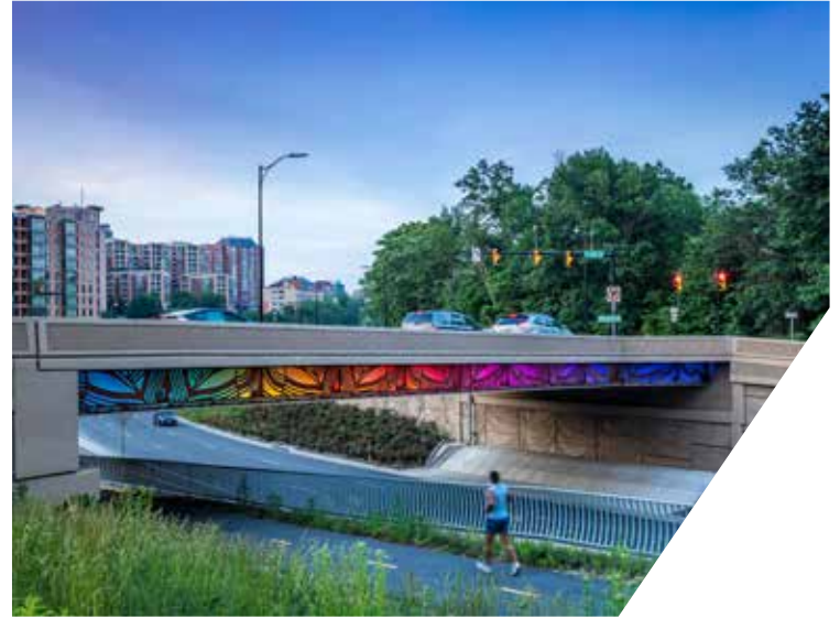
Arlington Boulevard Bridge, Vicki Scuri
